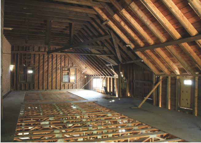
Stabalization of Carriage House Interior.
