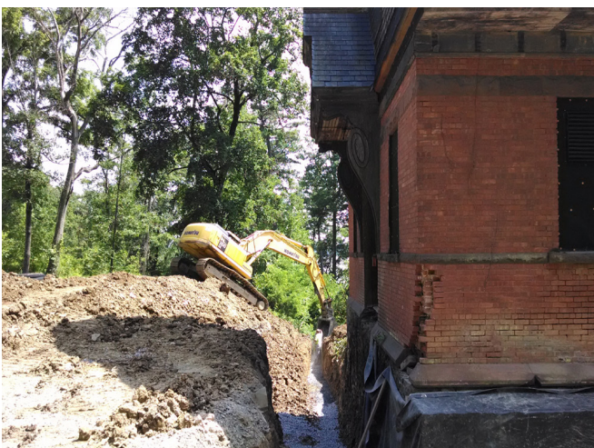
Carriage House Foundation Work.
