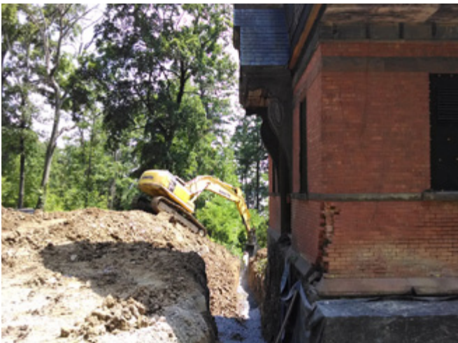
Carriage House Foundation Work.
