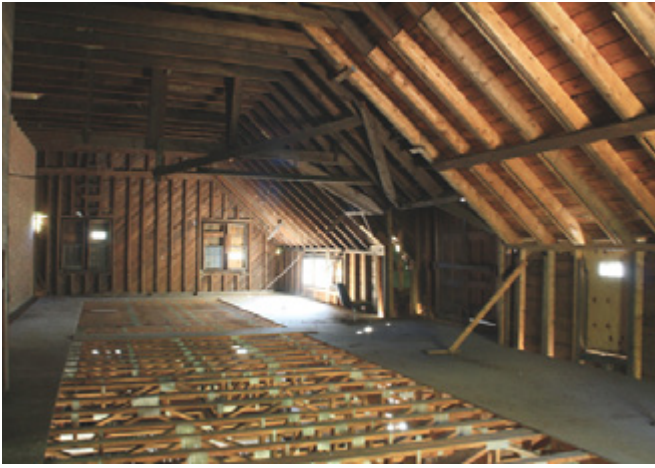
Stabalization of Carriage House Interior.
